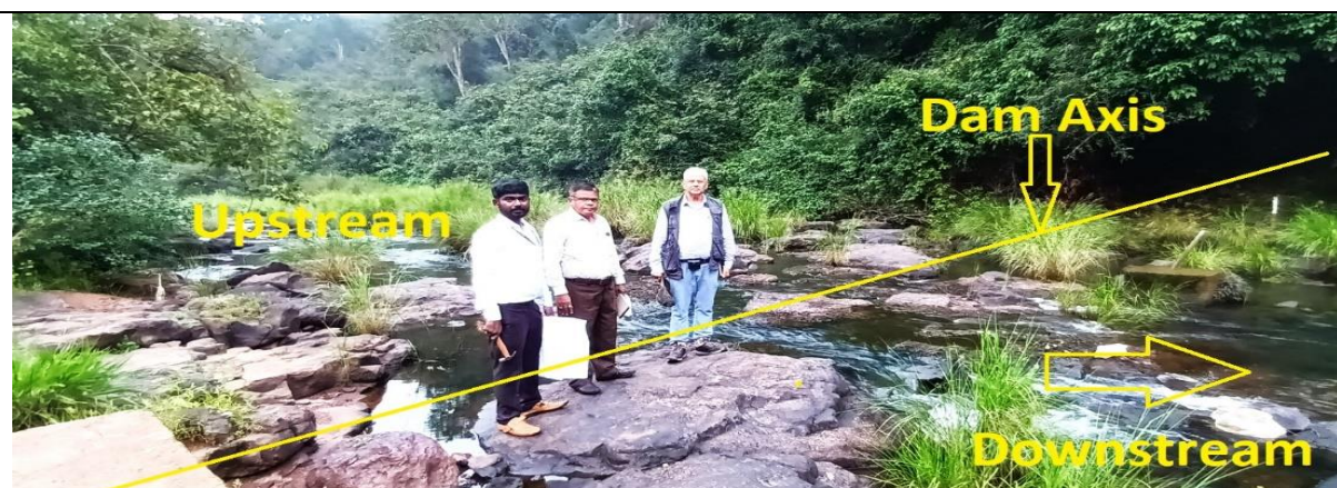
Figure 5: View of Dam site on Kalasa Nala exposed with basalt rock in the nala bed.
